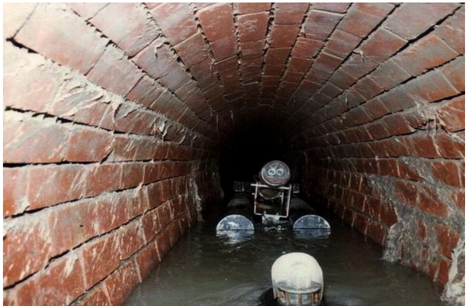
Peter's stereoscopic camera in a Melbourne brick ovoid conduit – early 1970's
